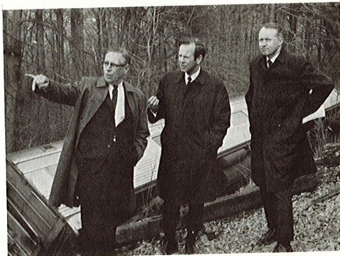
Rep. Brock Adams (D-Wash.) (center) visits the scene of the derailment of SCL's Gulf Coast Special on RF&P tracks outside Alexandria, Va., which killed three passengers. Mr. Adams is accompanied by Federal Railroad Administrator Reginald Whitman (left) and FRA Congressional Liaison Officer Donald Deuster. After viewing the wreck, Rep. Adams said that good rail safety laws could have prevented this accident and called for prompt action by the House on the Senate-passed rail safety bill.
